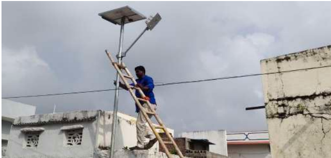
▲ Installation of solar-powered street lights
