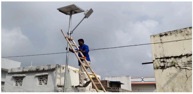
▲ Installation of solar-powered street lights
